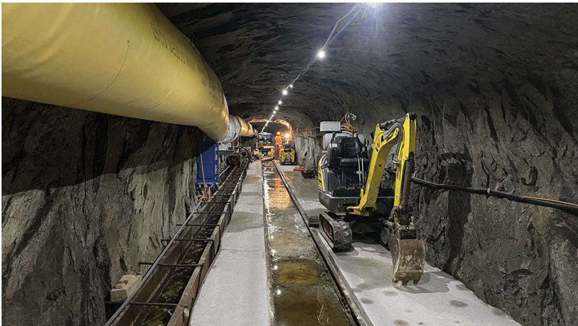
Construction work for the new earthquake physics testbed © BedrettoLab, 2022
