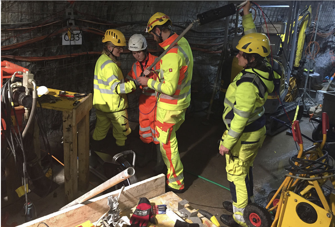
The installation of the monitoring network. © BedrettoLab, 2022
